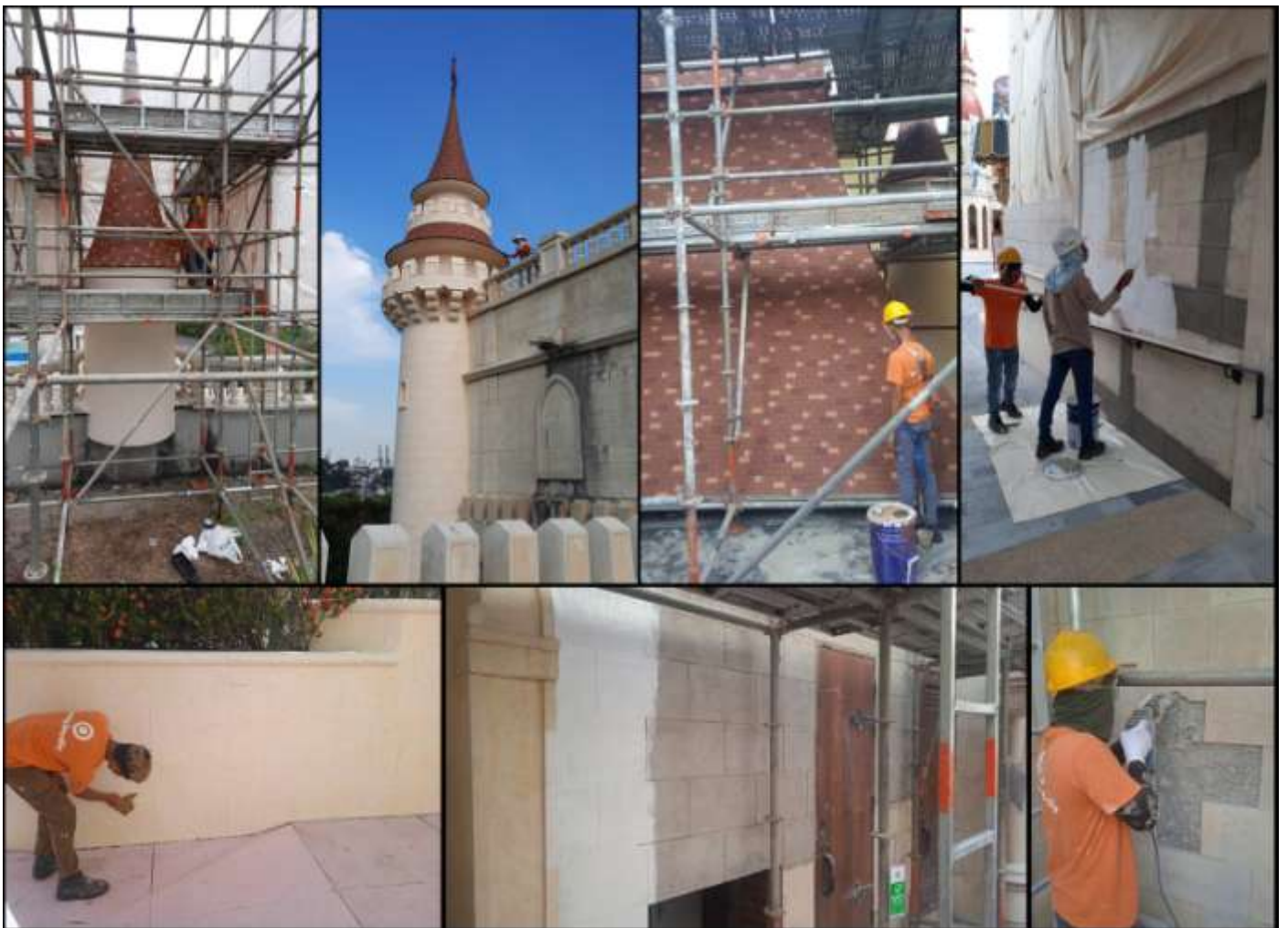
Façade RefurbishmentWork: Resorts World SentosaSG – Far FarAway
