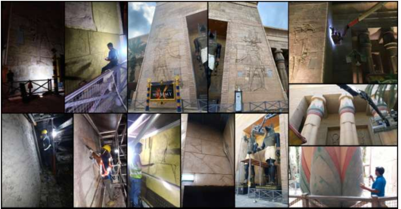
Façade RefurbishmentWork: Resorts World Sentosa SG– Return OfMummy
